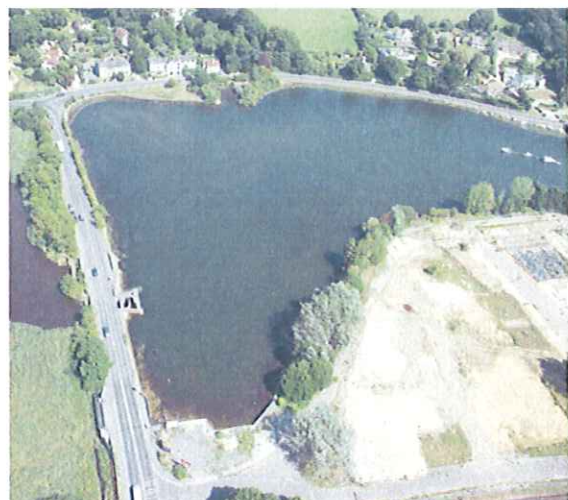
Aerial view of the current tidal flap on Bridge Road
